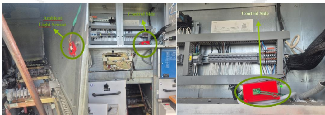
Figure 11. Field Installation of the Hardware
