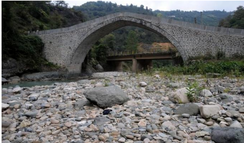
Fig. 1. An example of Historical Masonry Bridge in Giresun- Yağlıdere
